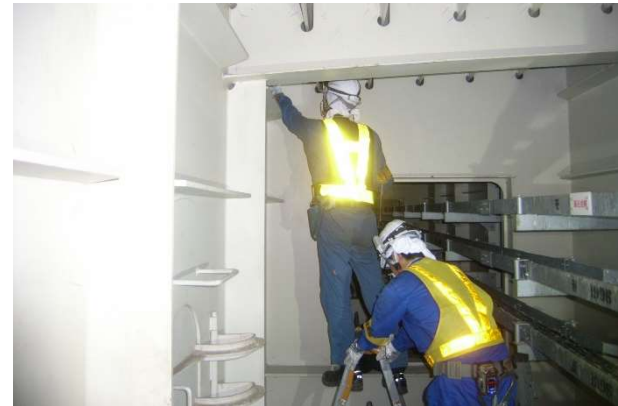
鋼箱桁内部の点検 Inspection of steel box girder inside
