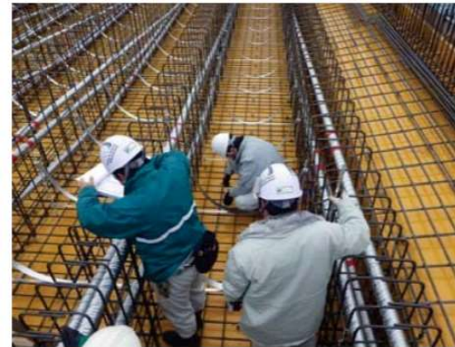
下部鉄筋 Lower reinforcement
