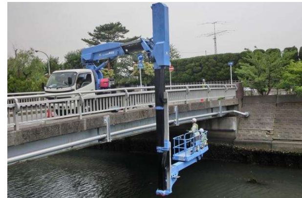
橋梁点検車 Bridge inspection vehicle
