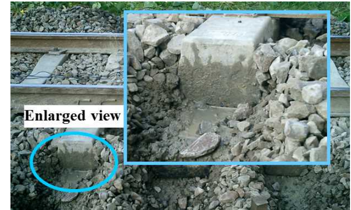
Fouled ballasted track in existing line
