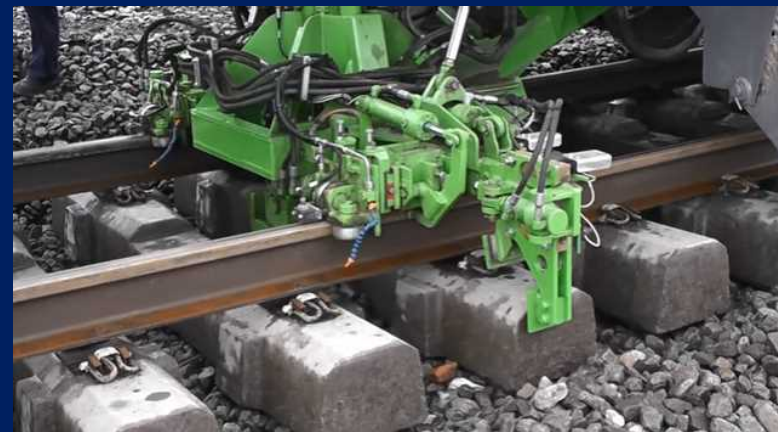
Winged sleepers implemented in a line
