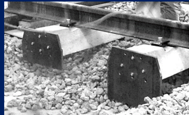
Buckling prevention plate
