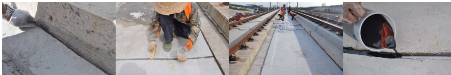
去掉水泥浮浆 Remove bleeding cement
