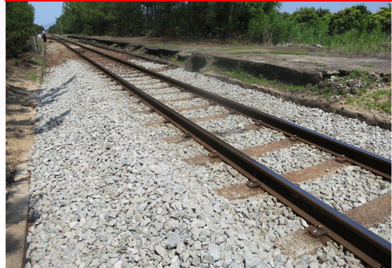
After roadbed improvement
