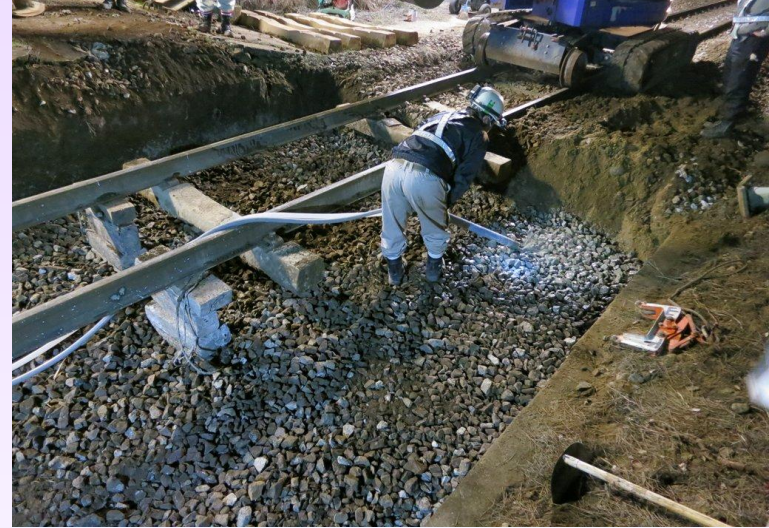
Injection of grout
