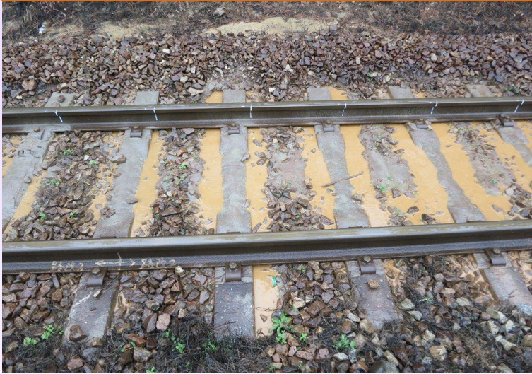
Before roadbed improvement
