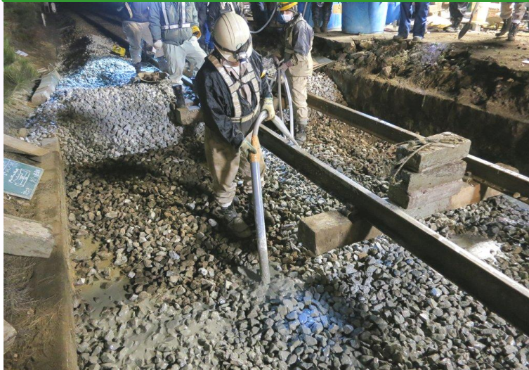
Injection of grout
