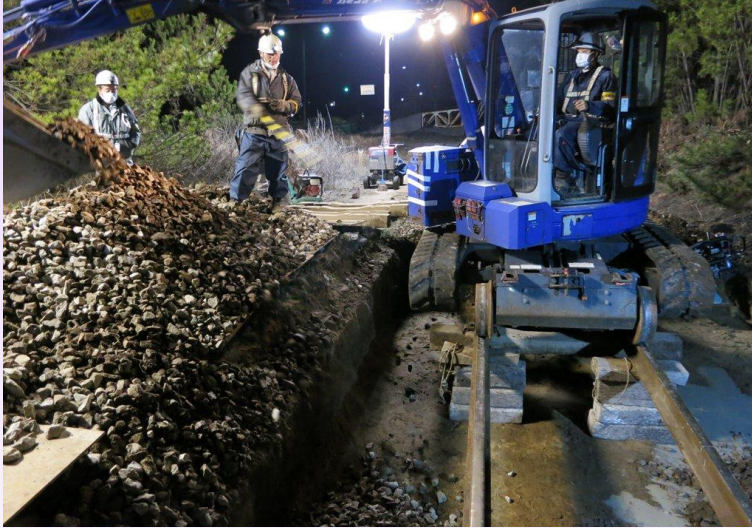
Laying degraded ballast
