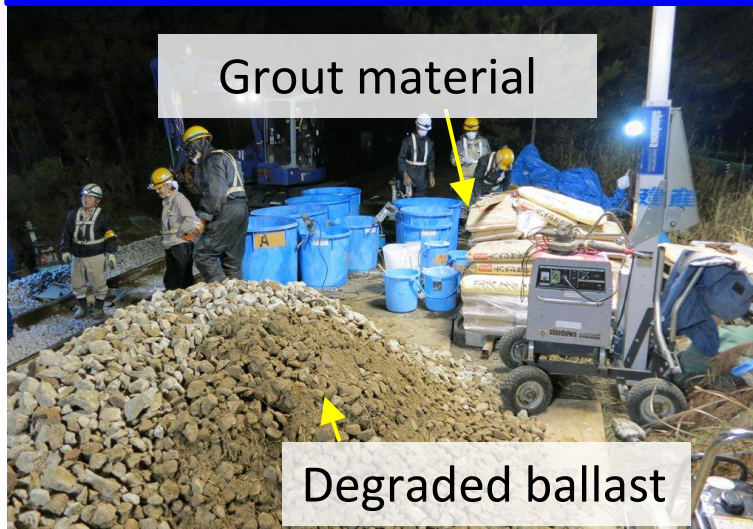
Degraded ballast
