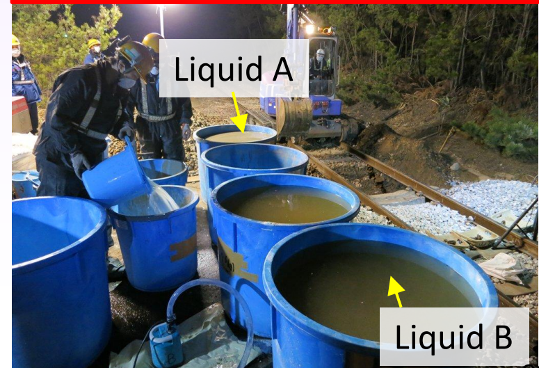
Preparation of grout
