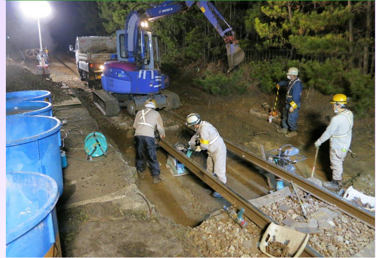
Excavation of ballasted track
