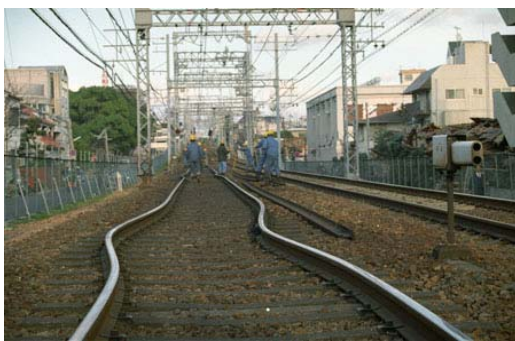
The buckling of longrail
