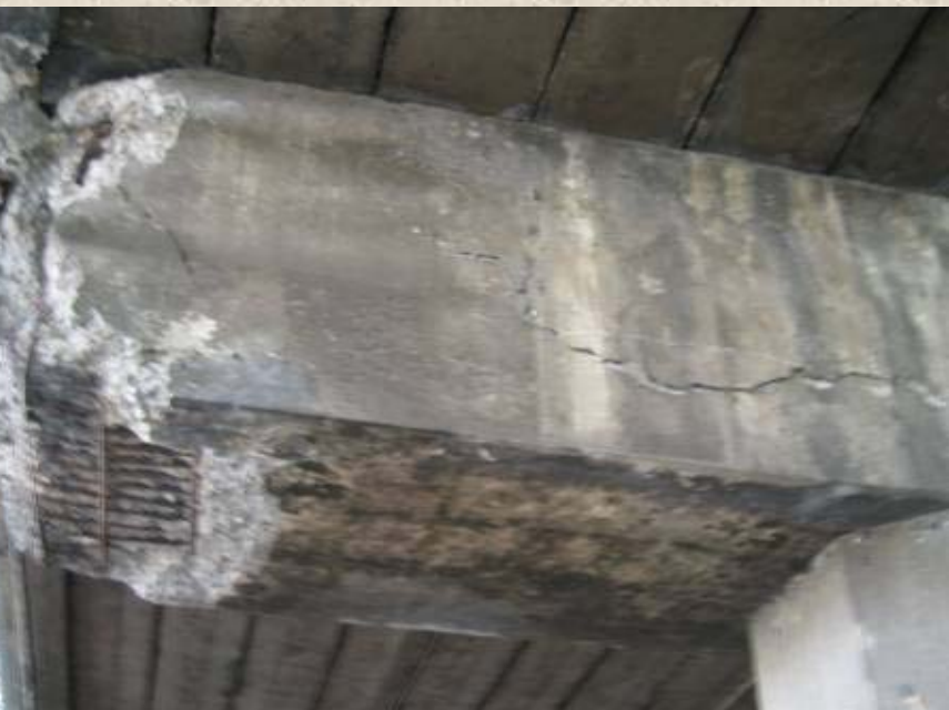
Carbonation induced steel corrosion
