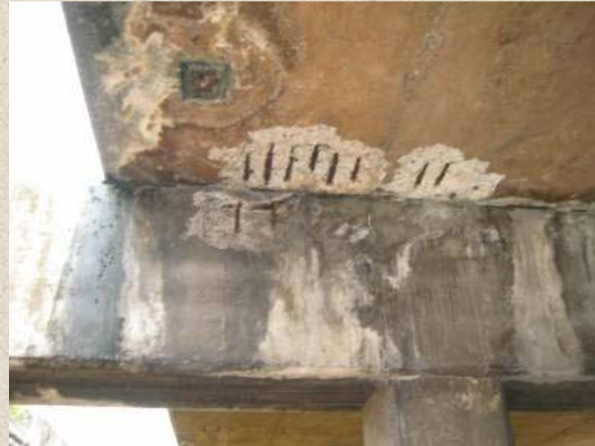
Carbonation induced steel corrosion
