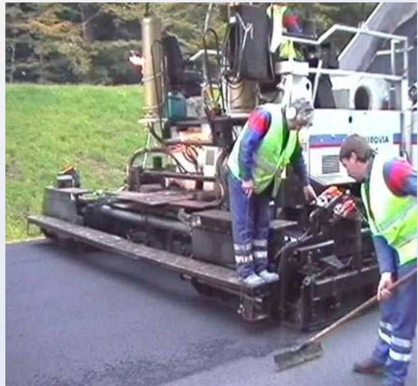
Machine-Paving
