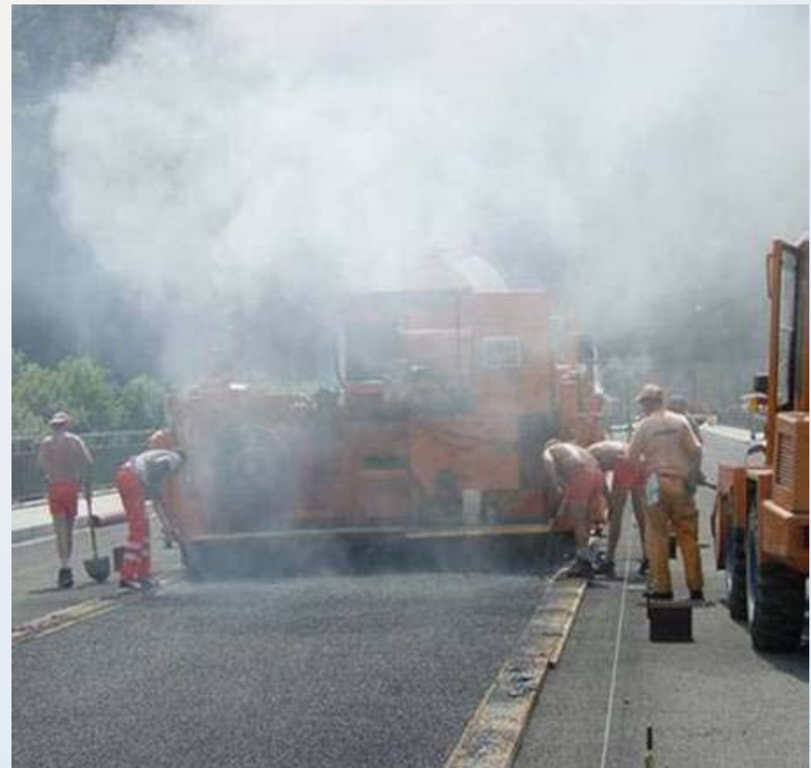
Machine-Paving
