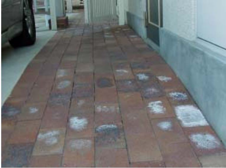
Efflorescence
