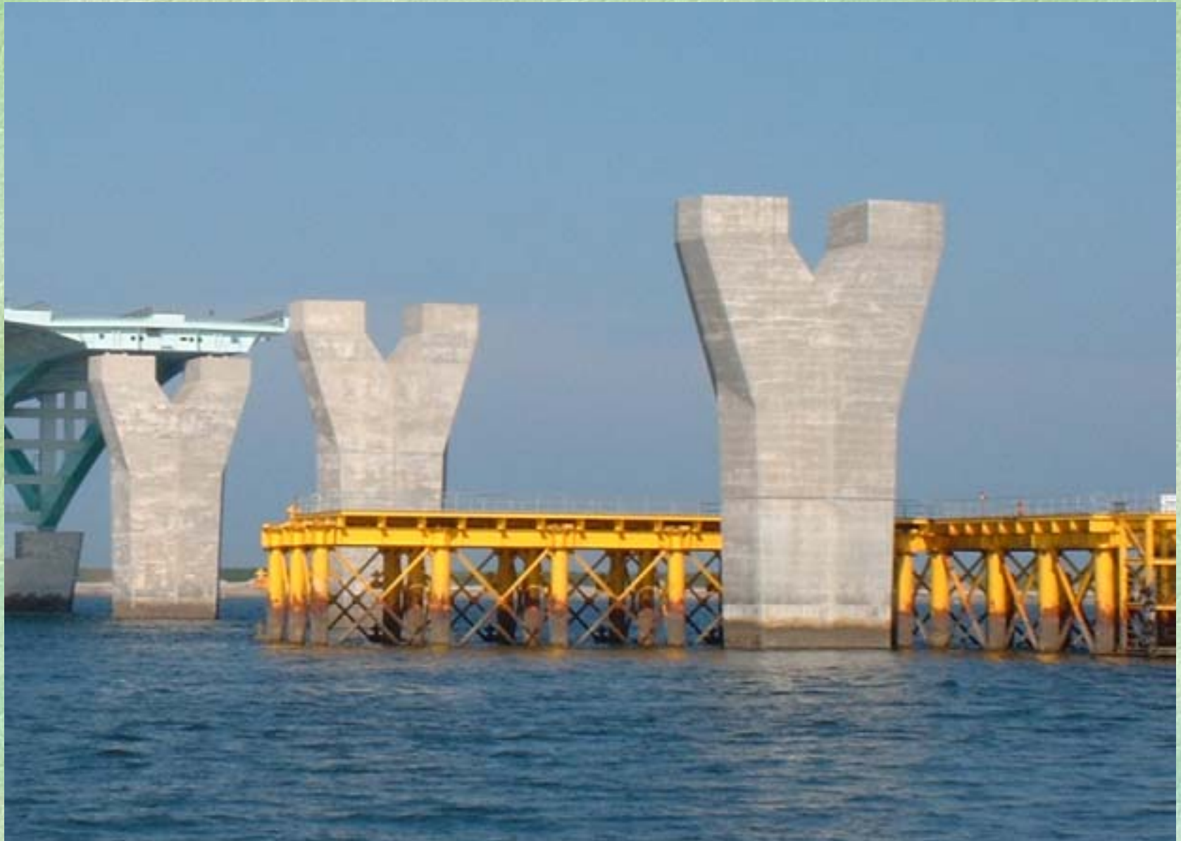
Piers of the Access Bridge
