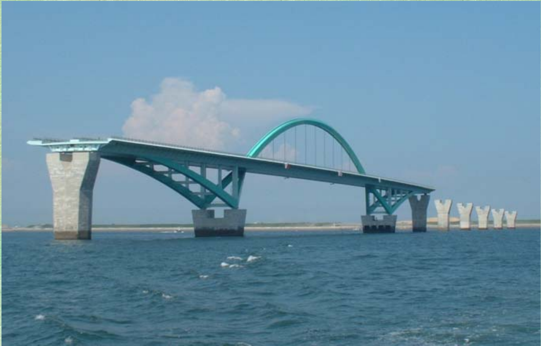
Main Bridge in the Access Bridge
