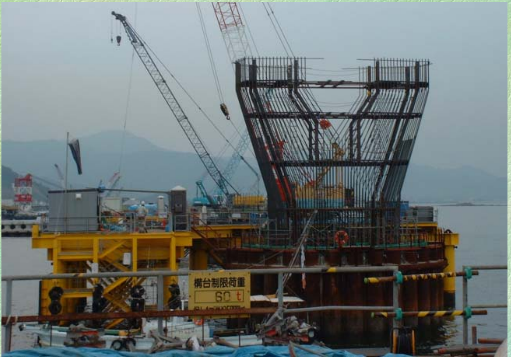
Arrangement Condition of Reinforcing Steel
