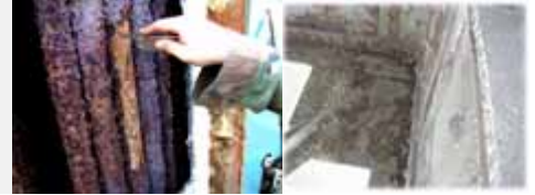
[ Carbonation at tunnel inside – T4 ]
