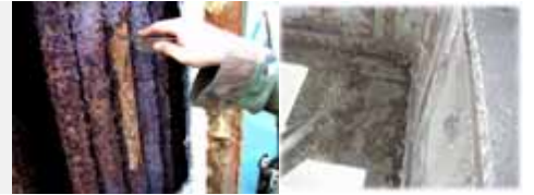
[ Carbonation at tunnel inside – T2 ]
