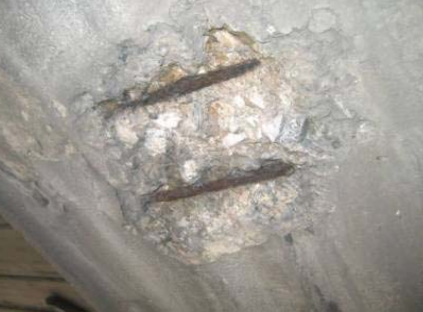
Carbonation induced steel corrosion
