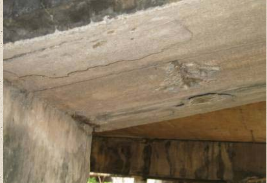
Carbonation induced steel corrosion
