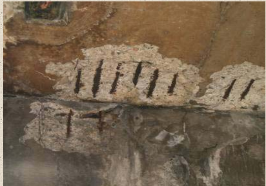
Carbonation induced steel corrosion
