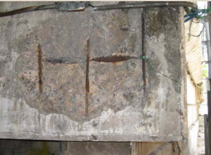
Carbonation induced steel corrosion
