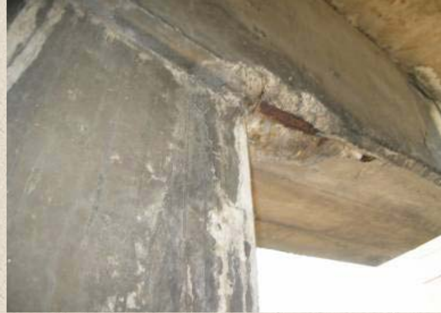
Carbonation induced steel corrosion
