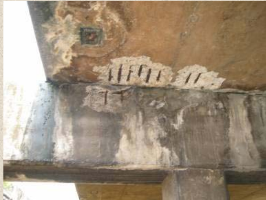
Carbonation induced steel corrosion
