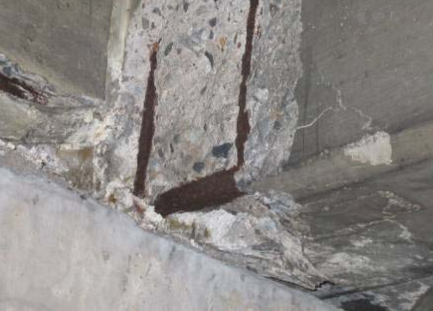
Carbonation induced steel corrosion
