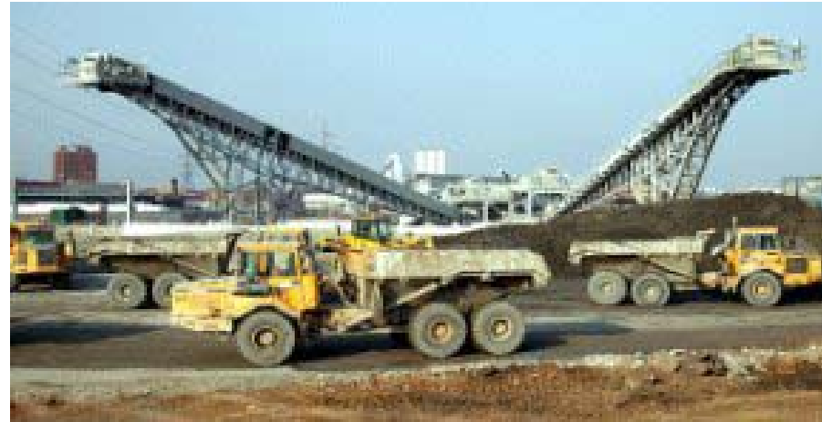
Spoil Disposal at Stratford
