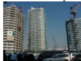
Job site of MM Towers
