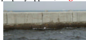
Proper mix-proportion & dense filling Otaru North Break Water
