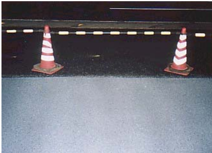
Application of photocatalyst \text{TiO}_2 on road
