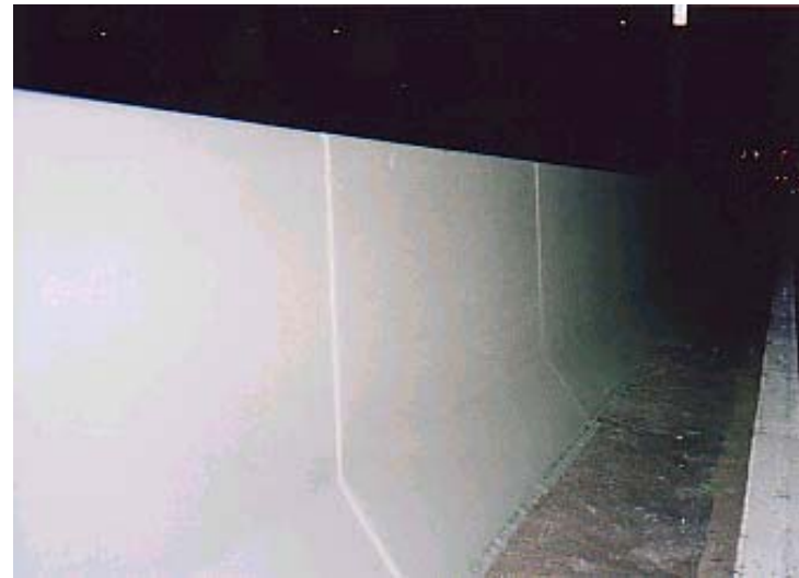
Application of photocatalyst \text{TiO}_2 on wall
