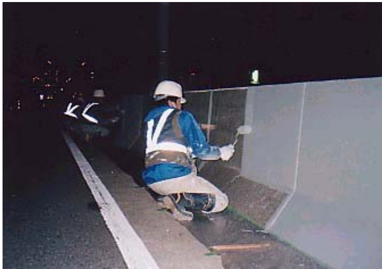
Application of photocatalyst \text{TiO}_2 on wall
