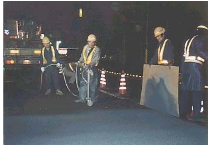
Application of photocatalyst \text{TiO}_2 on road
